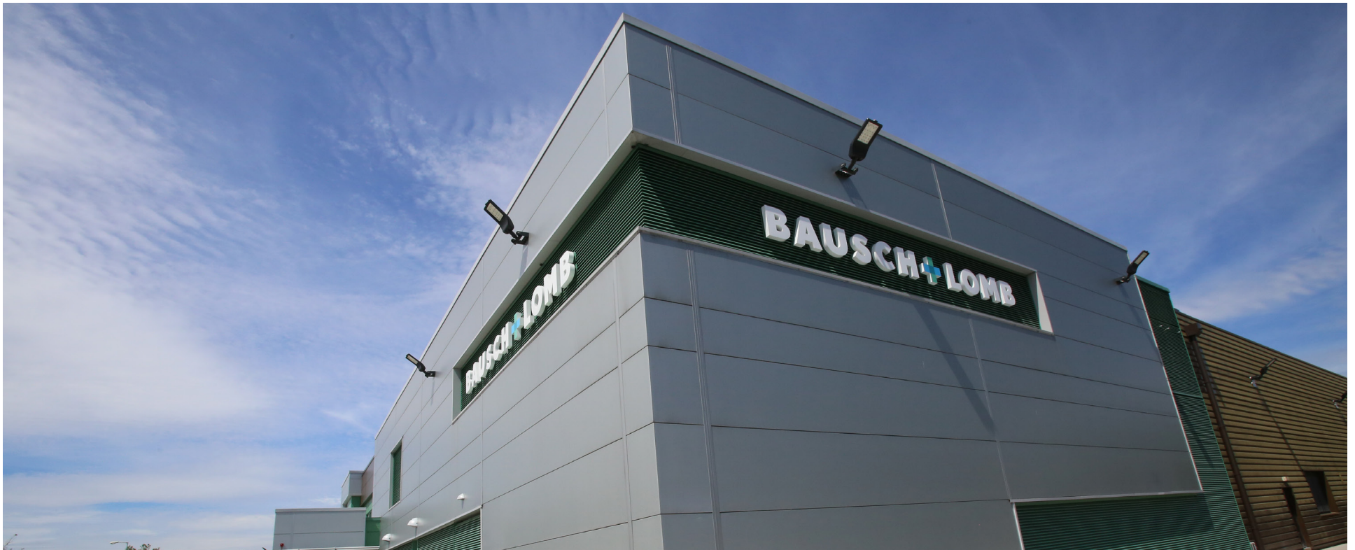
Bausch + Lomb's contact lens manufacturing plant in Waterford, Ireland.
