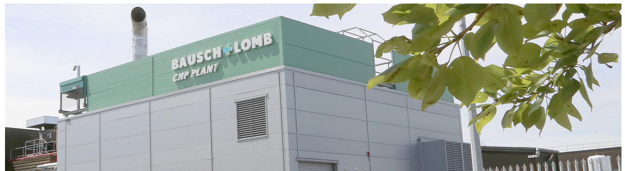
The combined co-heat and power plant (CHP) in Waterford, Ireland has improved energy efficiency and environmental impact.
